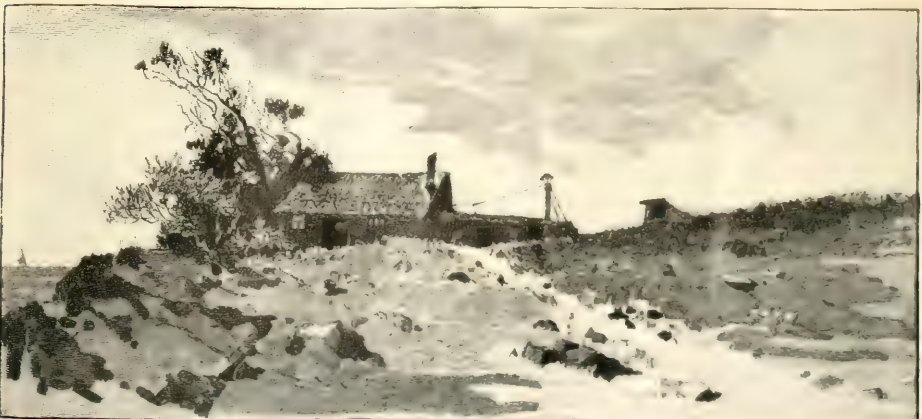
THE CRUMBLING COTTAGE.
